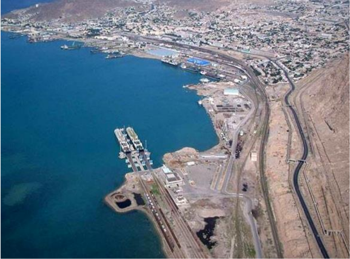
Turkmenbashi Port (Credit: www.dredgingtoday.com )
